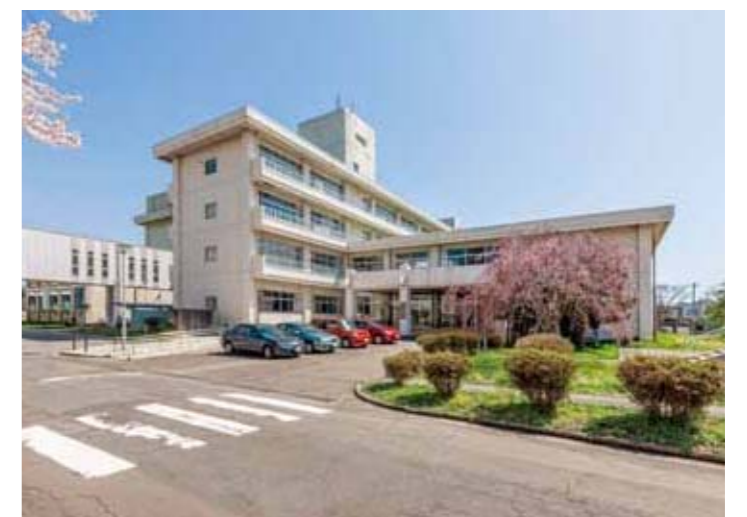
保健学科棟 Building for Health Sciences
